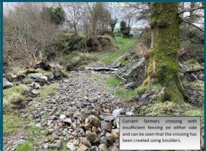
Barrier to fish migration and also river flow with narrowing the width of the river from approximately 6m to less than 1m in this point. Also collecting downstream flowing debris.
