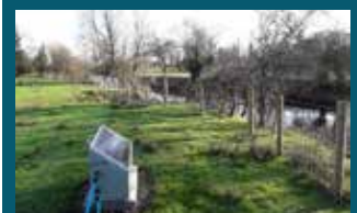
Fig. 4 Solar Pump on Arney River
